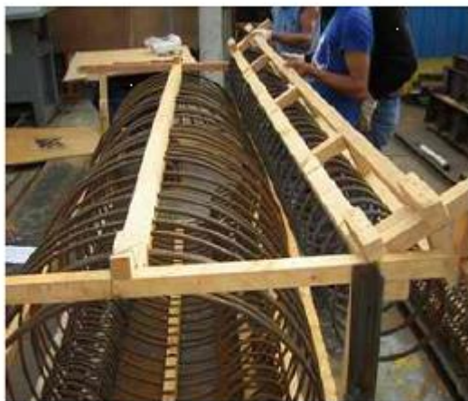
(c) Assembly of the upper two small spirals.
