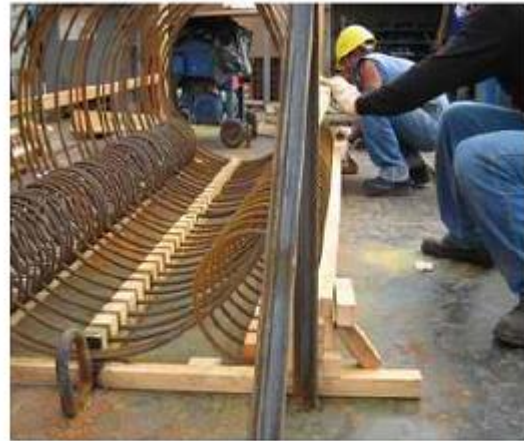
(b) Assembly of the bottom two small spirals.
