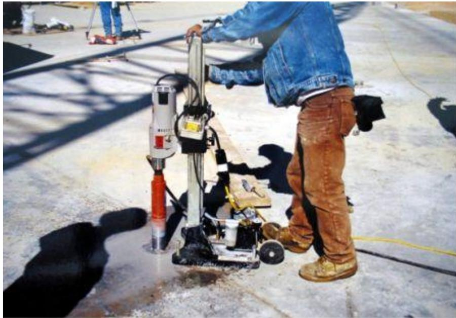
Fig. 11 Mat Foundation Drilling for Precast Cell Installation
