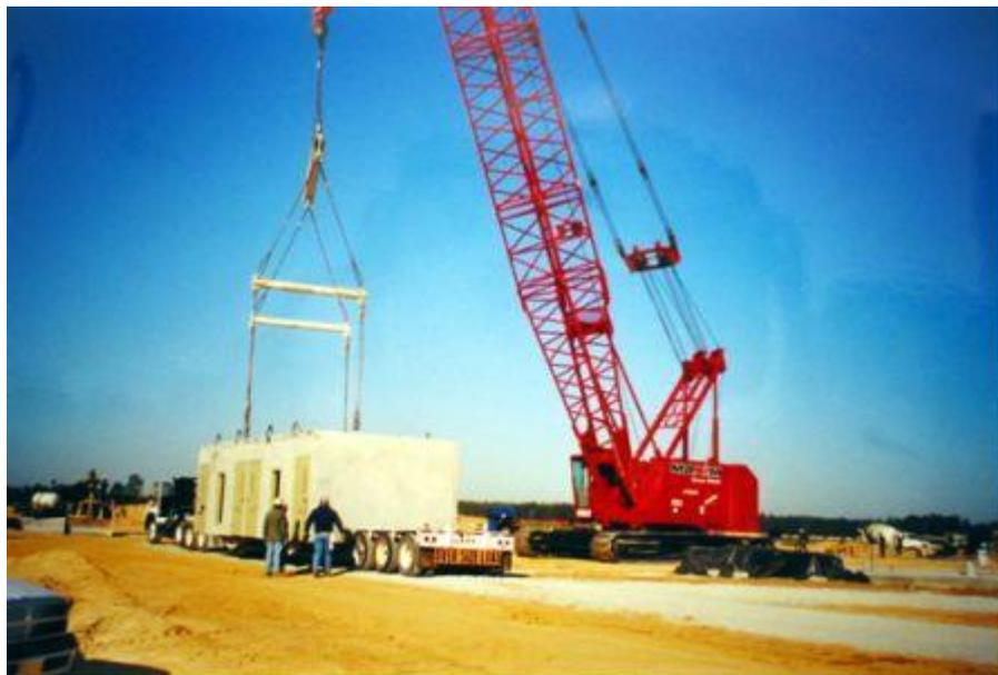
Fig. 10 Erection by Construction Crane
