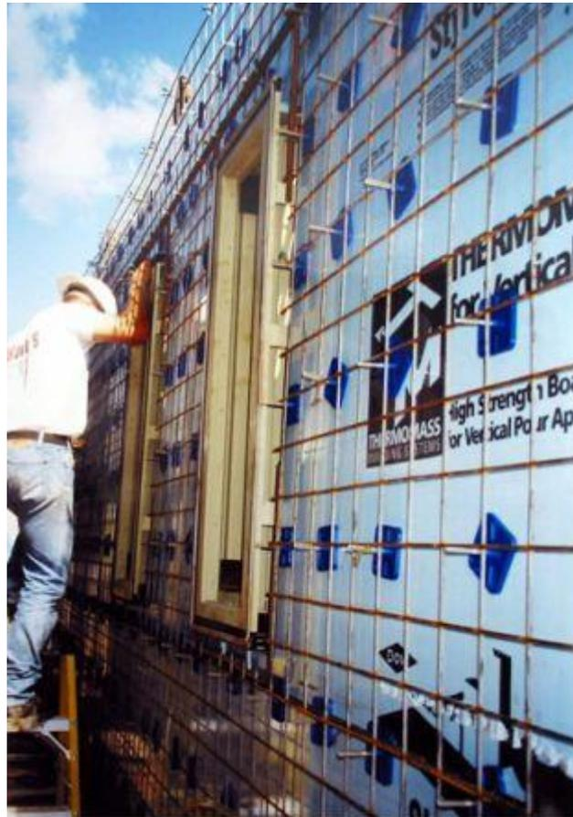
Fig. 8 Fabrication of Embeds Prior to Concrete Placing
