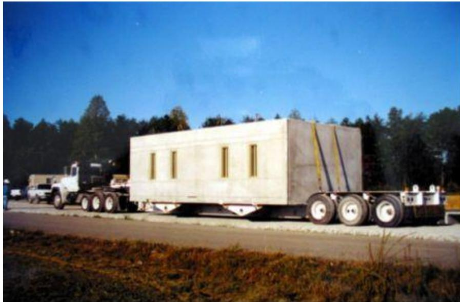
Fig. 9 Special Truck for Cell Module Transportation
